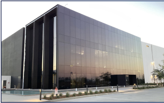
INSULATED GLASS: Facade - World Logistics Center (Moreno Valley, CA)
